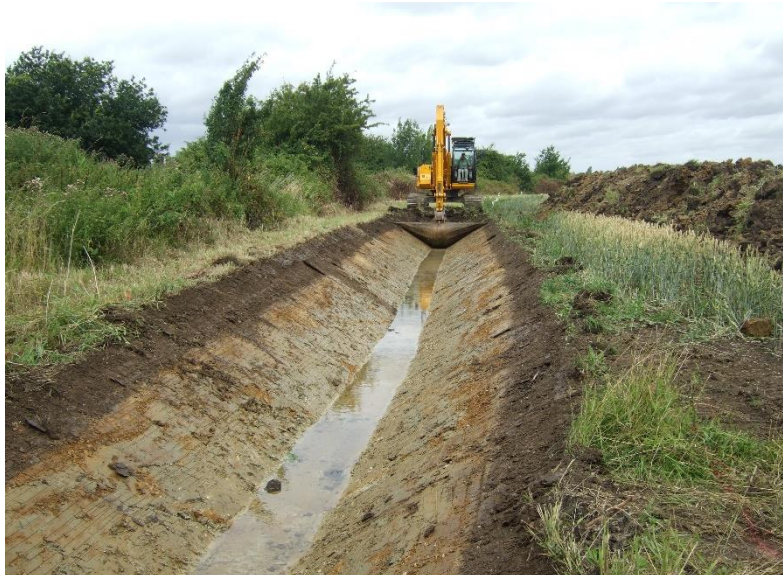
Figure 7-1: Completed action to create a new ditch near Eye Green to reduce flooding
